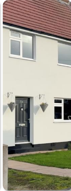
Fabric upgrades and insulation
