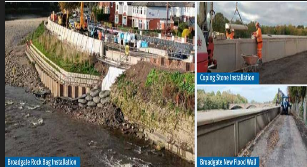
Preston & South Ribble Flood Scheme – Lancashire
