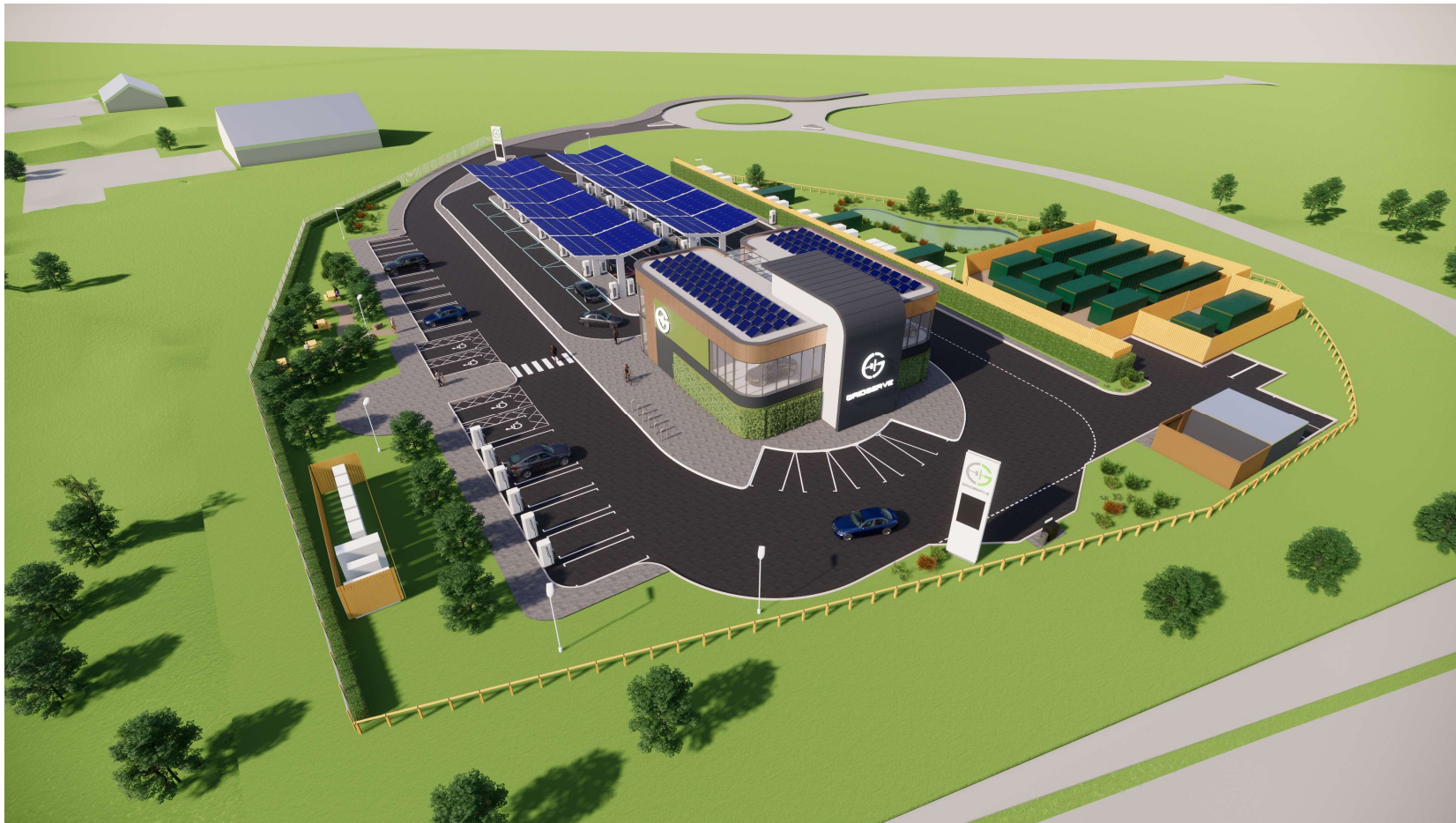
Overview of Braintree Electric Forecourt® including the multi-MW battery storage system in the green containers
