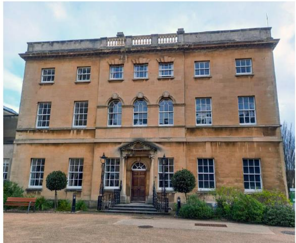
Figure 11: Air source heat pumps have been installed in an inconspicuous location to the right-hand side of the door and are barely visible on the front elevation of the Grade I listed building. © Historic England
