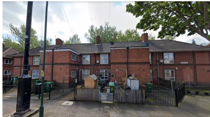
Mid-terraced Flat (First Floor) & End-terraced Flat (Ground Floor)
