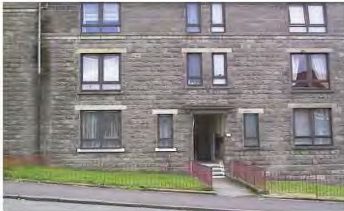
Typical block of flats for refurbishment
