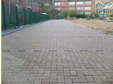
Sustainable Urban Drainage System (SUDS)
